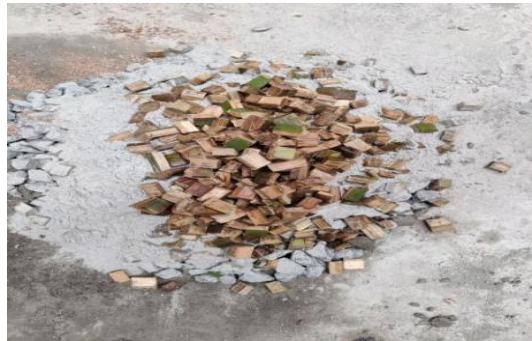
Bamboo chips replaced as aggregate to concrete mix
