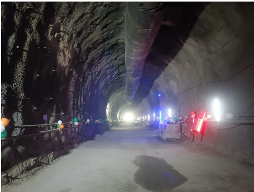
Fig. 4. Main tunnel and Ventilation
