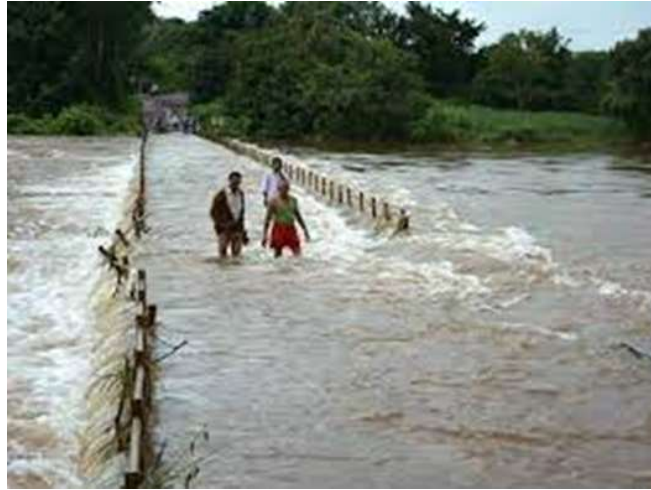
Fig. 1 : A typical bridge flooded with water
